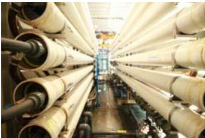
Installation de nanofiltration (2 installations comportant 15 caissons de 6 tubes de nanofiltration).
